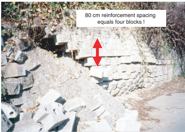
Figure 10. Typical example of failed GRS-MB retaining wall (sites 1 and 2)
