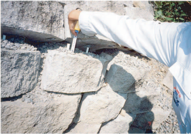
Figure 9. Typical example of connection pin seen in an opening between modular blocks (sites 1 and 2)
