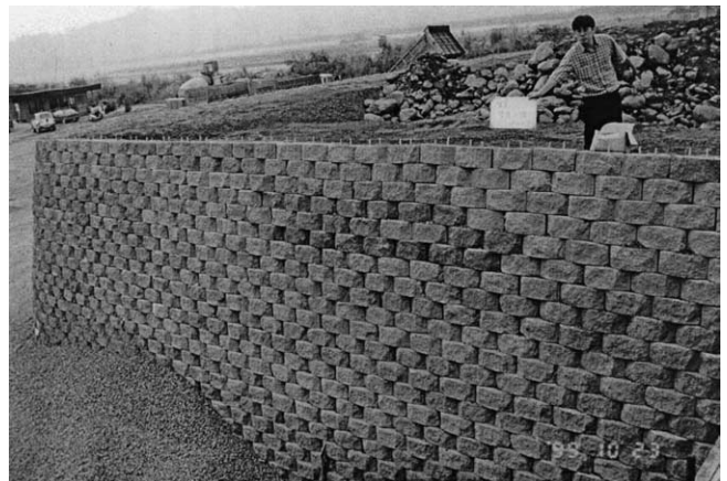
Figure 5. Undamaged GRS-MB wall at site 4
