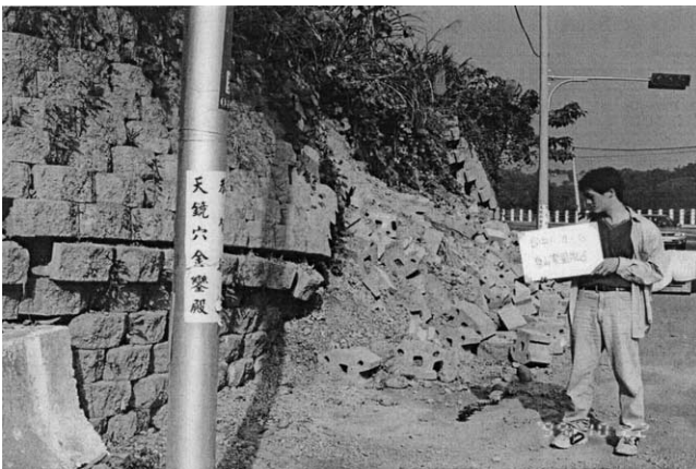
Figure 2. Collapsed GRS-MB wall at site 1
